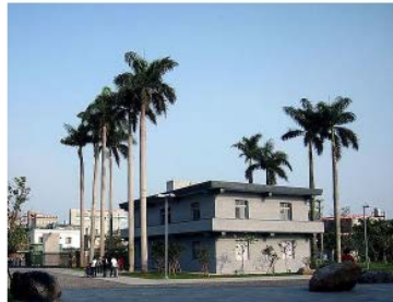
This is the building that was established in 1975, which was mentioned in the background part. And the building was named farmhouse (農禪寺). Afterwards, the building was restored, and Master Sheng Yan told the architect 6 words (空中花，水中月) → Water Moon Monastery (水月道場)
